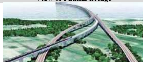
View of Padma Bridge
